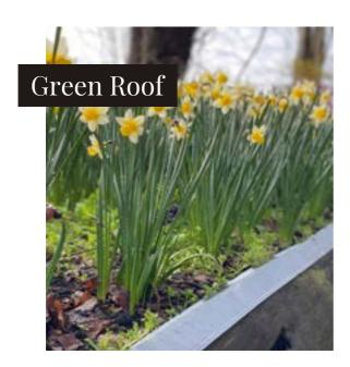
This specially constructed roof has a thick rubber membrane lining and is topped with several inches of soil allowing us to have a fabulous rooftop display.
